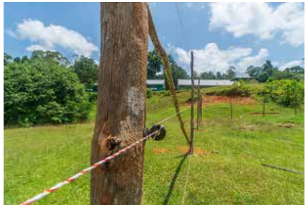
We helped the Berdiri Foundation build an electric fence to stop wild pigs from feeding on the vegetation needed by the conservation center's elephants. Now, the critically endangered Sumatran elephants will be able to roam inside their protected home.
