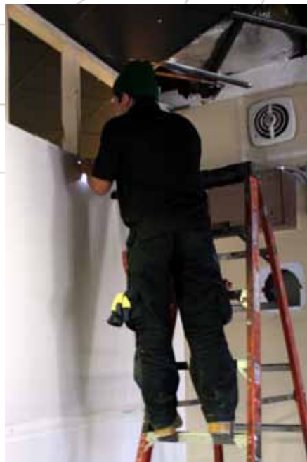
L.J. Wethey installs drywall in the Life in the Cold building. Our Operations crew took care of many major projects in the renovation of this four-building complex, from building walls to updating the plumbing.
